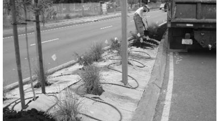
Sheet mulching site is ready for planting.
